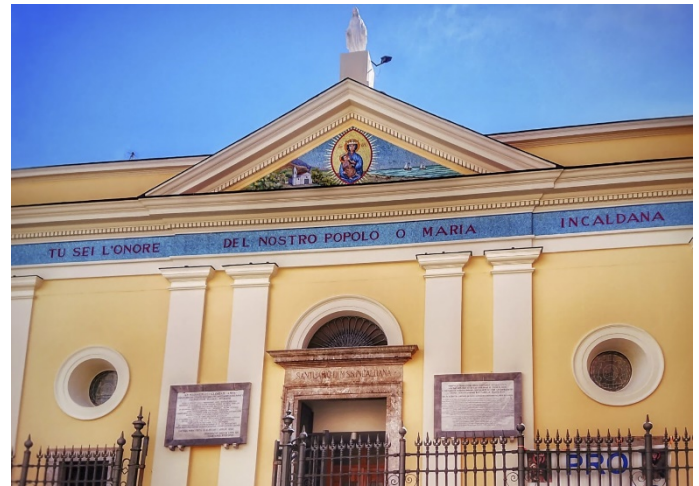
Fig. 9. Basilica Minore di Maria SS. Incaldana, external façade after restoration work (Ph: Angelo Razzano).
