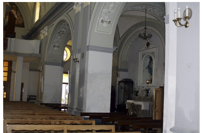
Fig. 2. Basilica Minore di Maria SS. Incaldana, left nave before restoration work.
