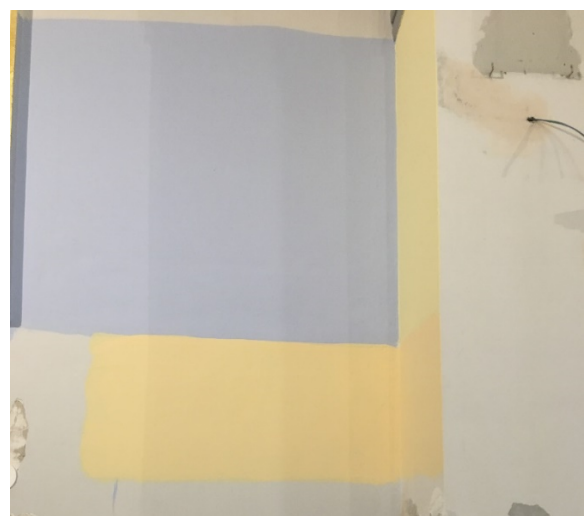
Fig. 7. Basilica Minore di Maria SS. Incaldana, testing of the new colors for the superintendence approval.
