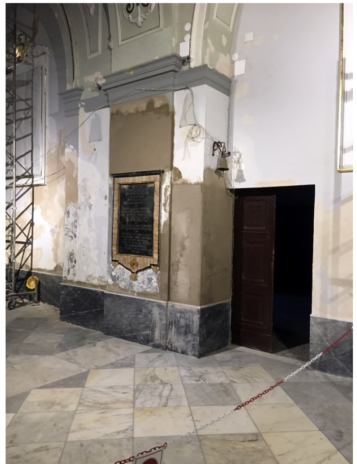
Fig. 4. Basilica Minore di Maria SS. Incaldana, right nave during restoration work.
