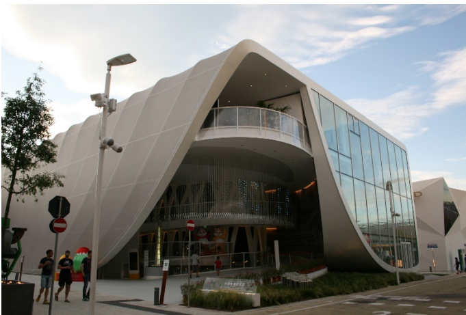
Fig. 1. China Corporate United Pavilion of Expo Milano 2015 in Italy, designed by the Architectural Design and Research Institute of Tongji University Ltd. A typical example of whitish textile surface. Photo © Alessandro Premier.
