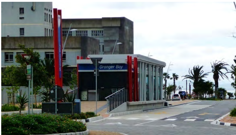
Figure 3: MyCiti station, Granger Bay station at Cape Town stadium, Cape Town Source: Hugo, 2012: Own photograph
