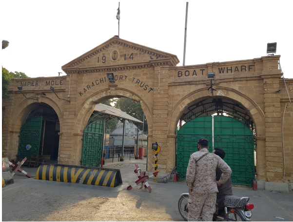
FIGURE 8. Karachi port Boat wharf entry gate.
