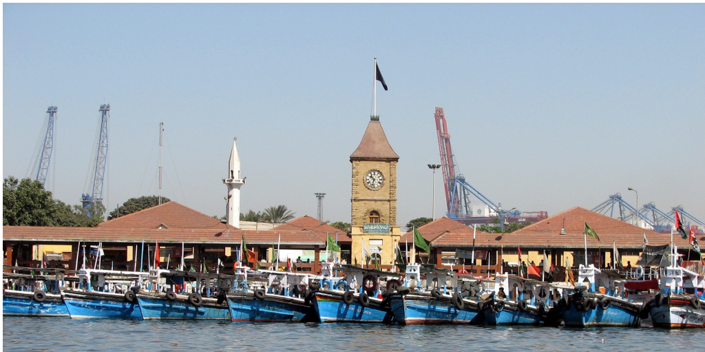
FIGURE 2. Boat Basin, Passenger Wharf Karachi port.
