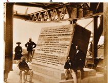
Karachi Harbour breakwater 1874 image from KPT archives
