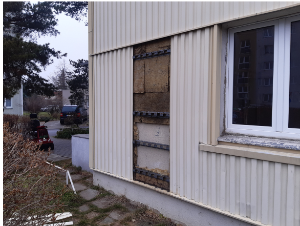
FIGURE 1. Building facade under reconstruction.
