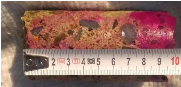
FIGURE 5. The carbonation depth of concrete at the places where the render was missing - sample selected from the measurements performed in 2018 (Bridge in Sládkovičovo).
