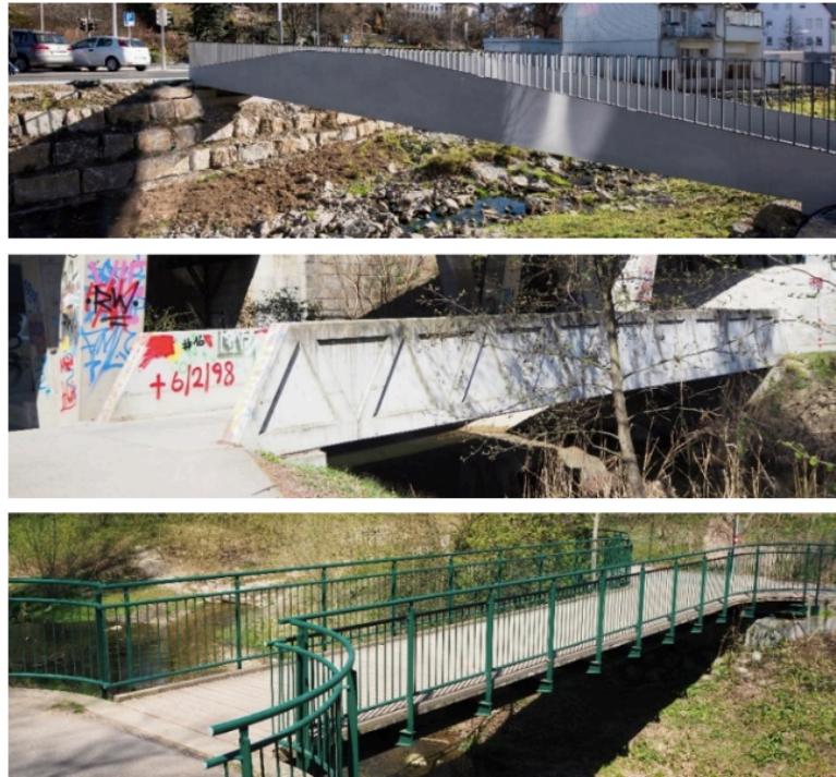
FIGURE 8. Pedestrian bridge examples, from top to bottom: B1-CCB (solidian GmbH), B2-RCB and B3-SB (Mathias Hammerl).
