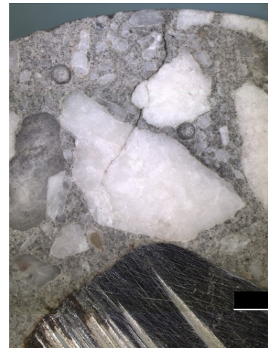
FIGURE 6. Microscopic image of polished cross section from a cracked specimen reinforced with CS bar, after corrosion initiation.
