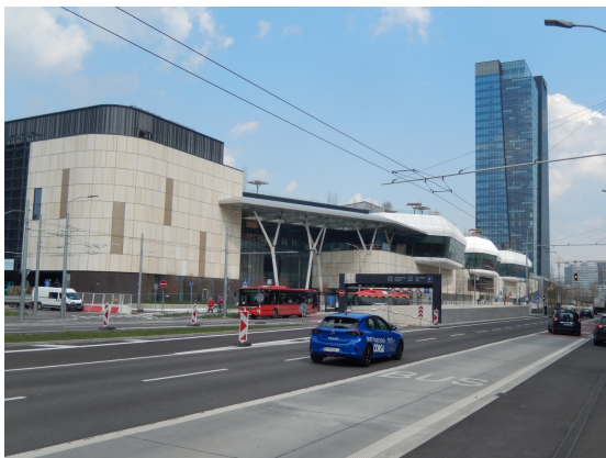
FIGURE 3. View of the completed area of the bus station.
