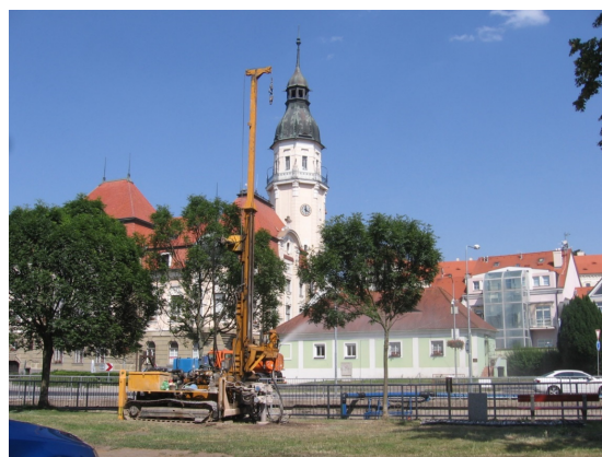
FIGURE 3. Groundwater monitoring well realisation, to the left in the background the historical building of Bílina city hall.
