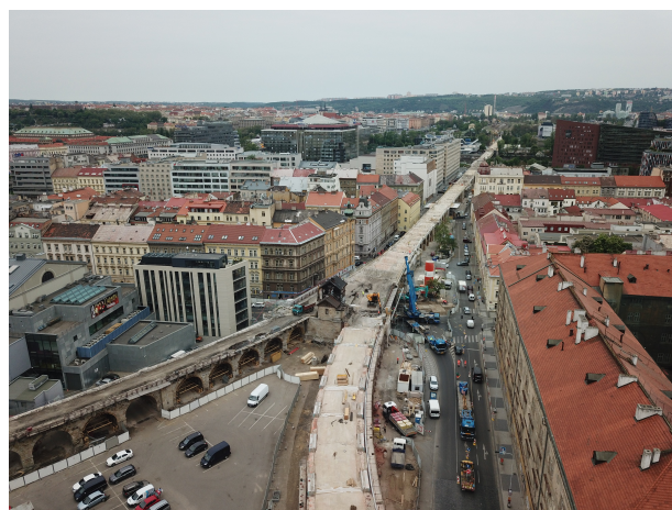
FIGURE 1. Bird's-eye view of the Negrelli's Viaduct during the reconstruction.
