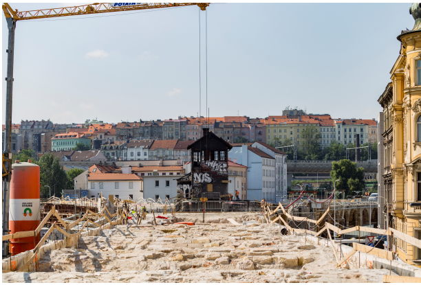
FIGURE 2. View of the exposed sandstone arches of the viaduct.
