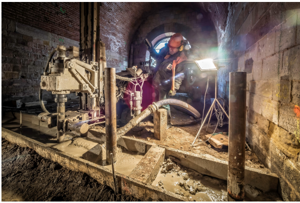
FIGURE 3. Special foundation works at the former custom house.
