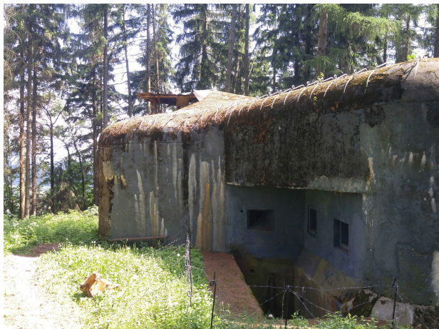
FIGURE 1. Sampling site: bunker No. T-S-20.
