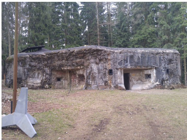
FIGURE 2. Sampling site: bunker No. T-S-19.
