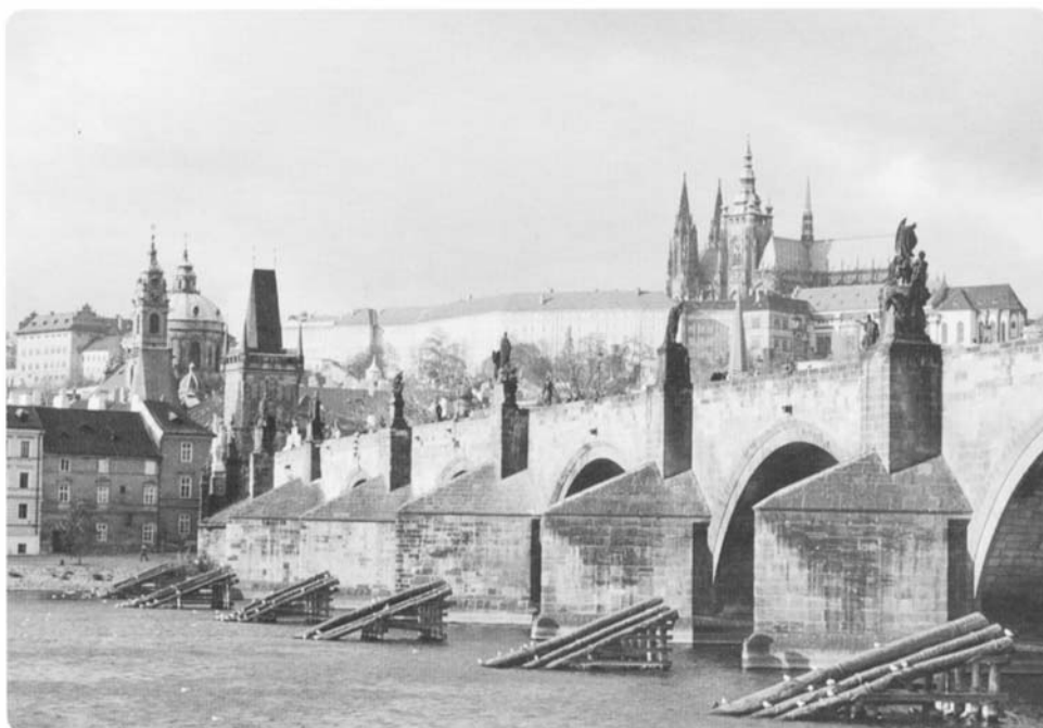
Photo 1: Charles Bridge in Prague
