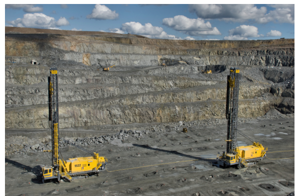
FIGURE 1. Two AtlasCopco drilling machines (Pitviper-351) in the process of drilling targets in a bench.
