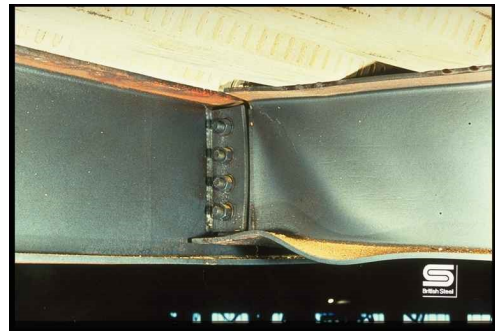
FIGURE 1. Shear buckling and bottom-flange buckling in Cardington fire test [4].
