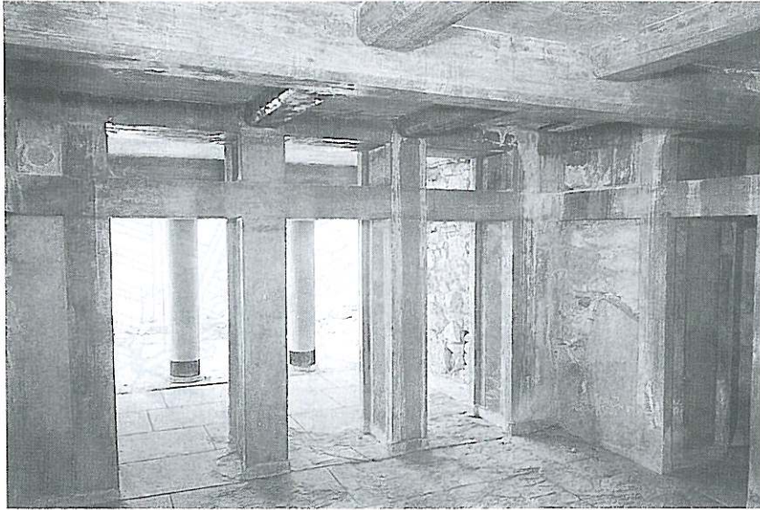
Fig. 5. Part of a Minoan villa at Knossos. The statically and dynamically daring style is counterbalanced by the extensive and sophisticated use of wood.
