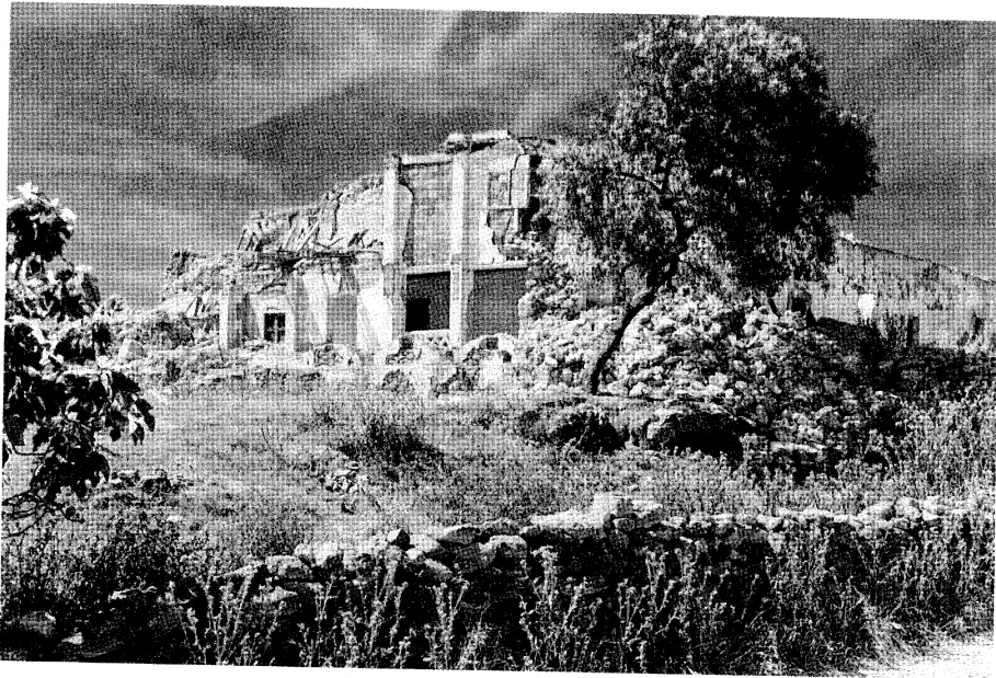
Photograph 1. Example of a construction that was almost-completely destroyed by the earthquake of May, 26, 1994 (Douar of Tafensa). Location in figs. 4 and 5.
