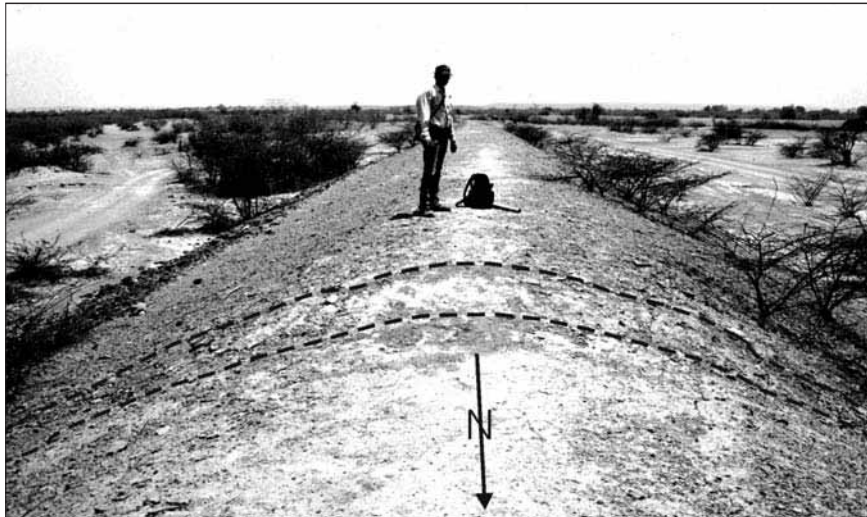
Fig. 8. Thrust scarp (between dashed lines) crossing the axis of a north-south-trending, 2.3 m-high earth dam (dike), at 23^{\circ}34.705'N , 70^{\circ}24.140'E . The scarp reaches a maximum height of 20 cm at the dam crest, and is slightly higher on the western side of the crest than on the eastern side, implying a small component of dextral slip in addition to north-directed thrusting. The apparent dip of the fault as it ascends the east side of the earth dam is 36^{\circ} south.
