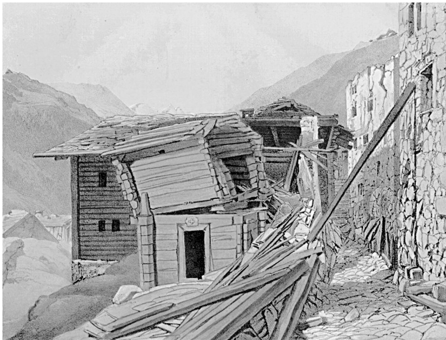
Fig. 1. Realistic drawing of an unknown artist from a typical building (Mazot) near Stalden/VS, damaged by the Earthquake of 25 July 1855 (in: Heusser, 1856).
